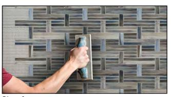
**Step 4** To achieve the flattest possible surface, lightly tap the sheets with a rubber grout float. Pay particular attention to the sheet-to-sheet intersections.
